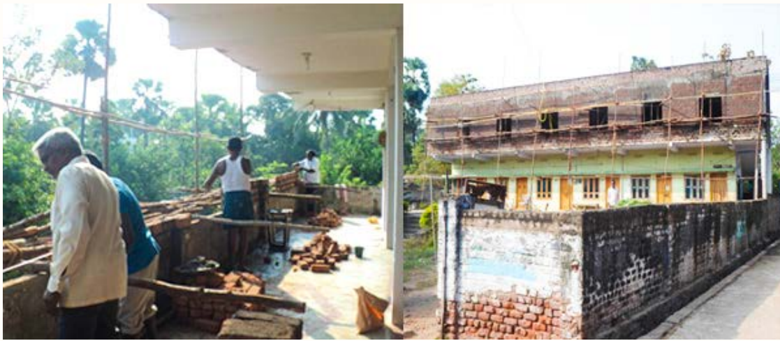
Construction is progressing
